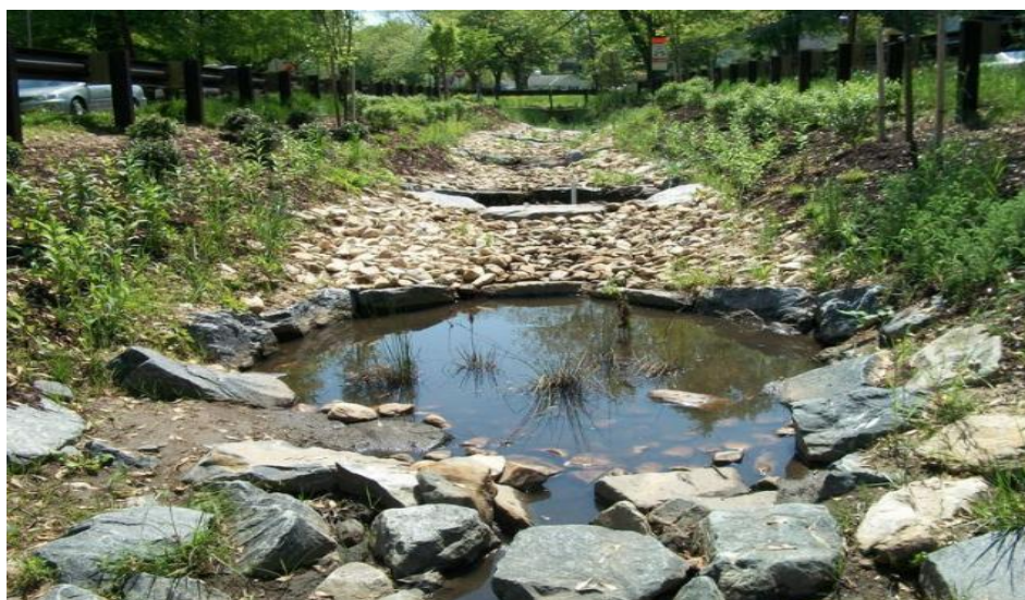
Figure 6.2 Loose Stone Check Dam (Source: Flickr Loose Stone Check Dam)
