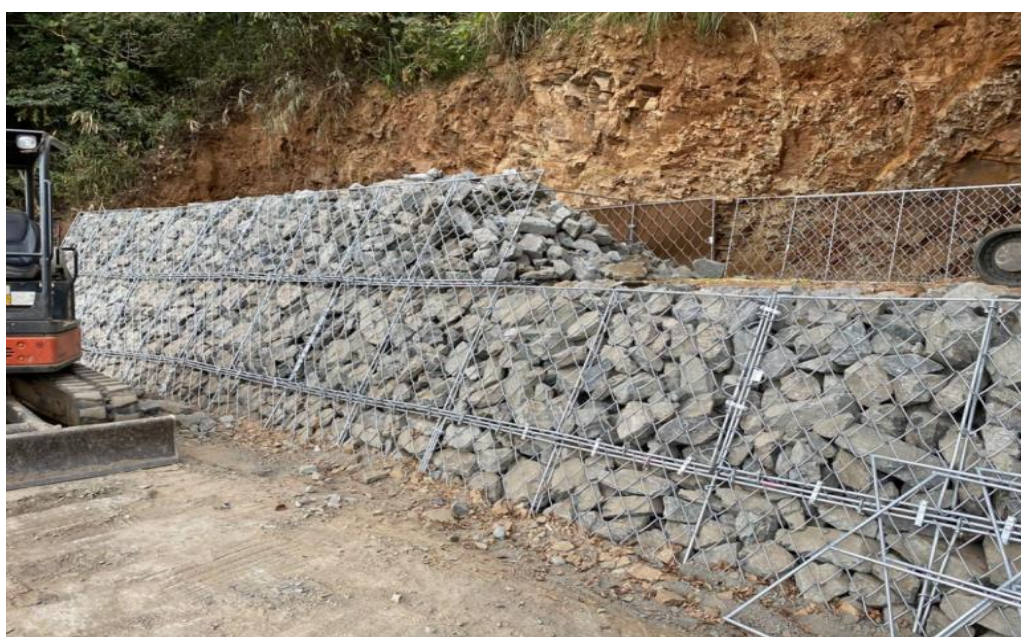
Figure 6.3 Gabion Check Dam (Source: Pinterest Gabion Check Dam)
